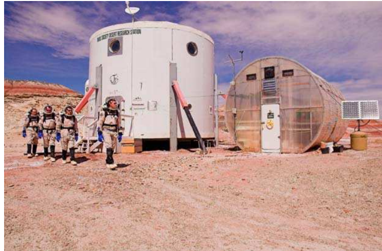
Fig.1.: The Mars Desert Research Station: the central Habitat has a diameter of 8m. In addition a solarpower station, a greenhouse and a small astronomical observatory complement the central infrastructure.
